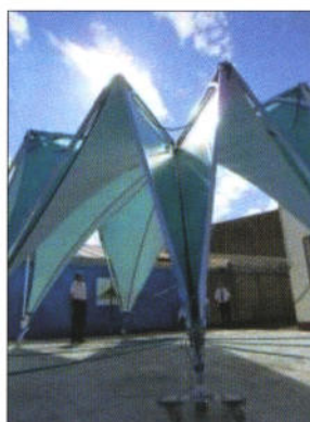
Figure 2: Contex-t demonstration of a foldable membrane construction. Involved partners: IASO – construction, Sioen – membranes, VUB - design.
